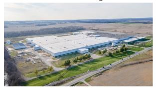
It is projected to process 145,000 bales of plastic film annually into 110 million pounds of recycled polyethylene. With FDA certification and a strong supply chain of retail film sources, SYNDIGO1 represents a significant leap forward in mechanical recycling infrastructure.
