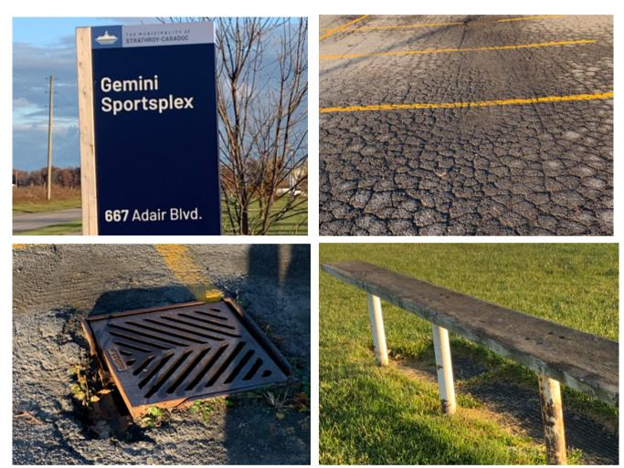
Parking lot lighting is in good condition, but the asphalt surface is only in fair condition, with numerous cracks and visible wear. Several catch basins are in poor condition, with approximately four requiring immediate repair to prevent further deterioration. Each catch basin repair is estimated to cost between \$4,000 and \$4,500. Overall, the parking lot's condition is rated as fair to good, pending these necessary repairs.
