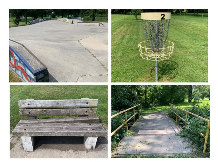
The bridge located in the park is in fair condition. Plywood has been installed in a few sections that now pose a trip hazard. Consideration should be given to replace the planks and to have the bridge inspected by a structural engineer. The cast in place concrete skatepark is in good condition with limited signs of cracking. The concrete should be monitored annually for signs of deterioration. Benches are noted to be in poor condition and should be replaced.
