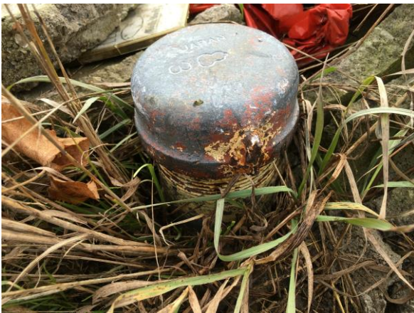
Photograph 5: Close-up of suspected filler pipe
