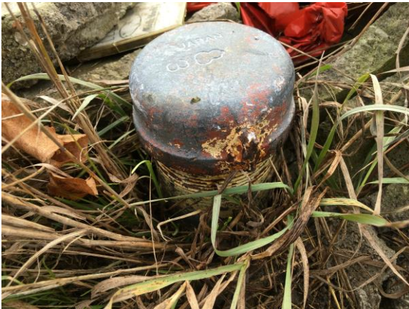
Photograph 5: Close-up of suspected filler pipe
