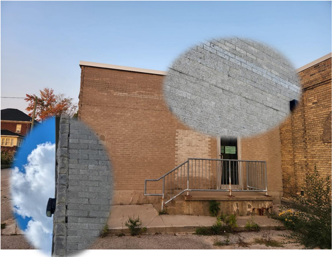
Step Cracking
