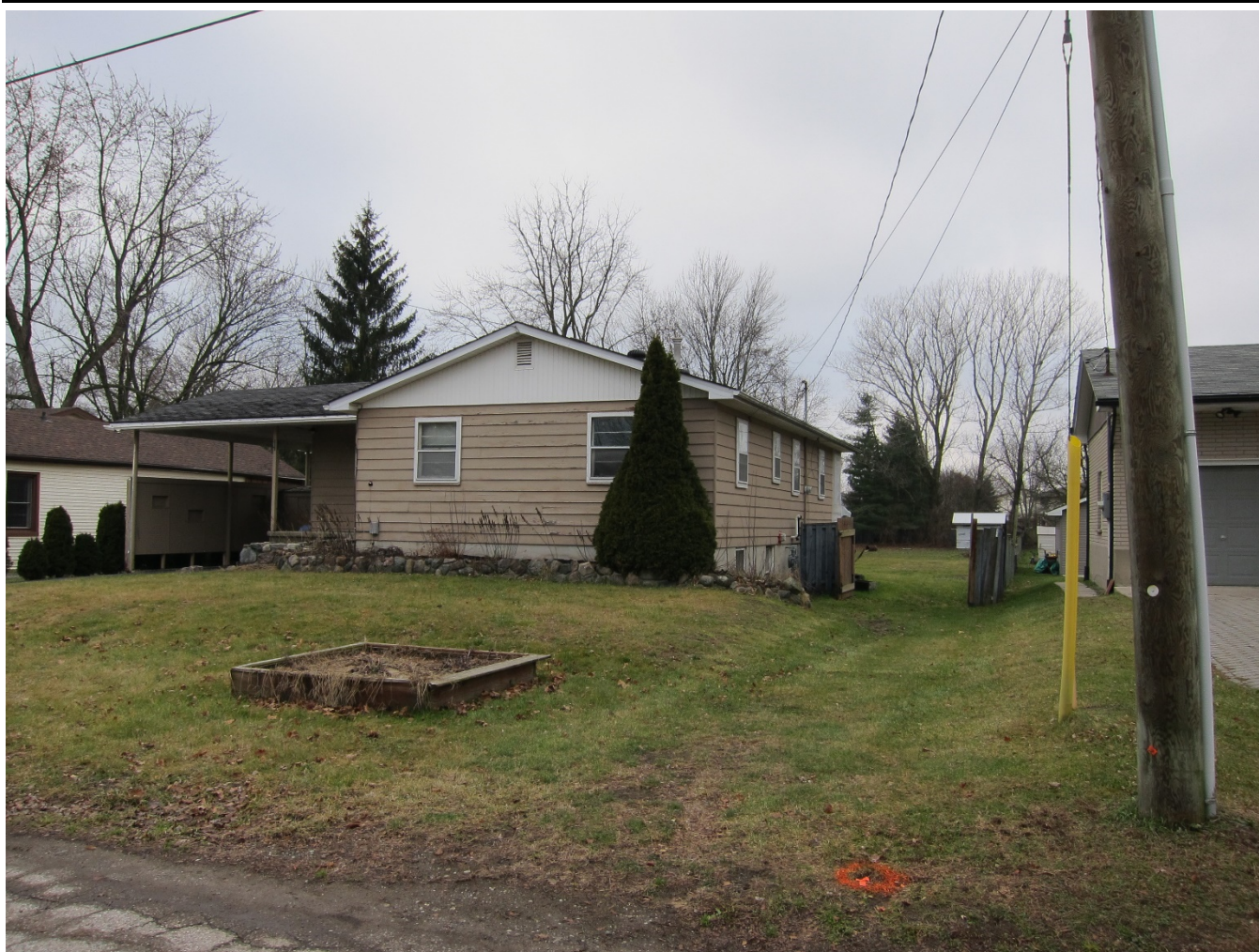
Photo #3: View of Subject Property looking southwest
