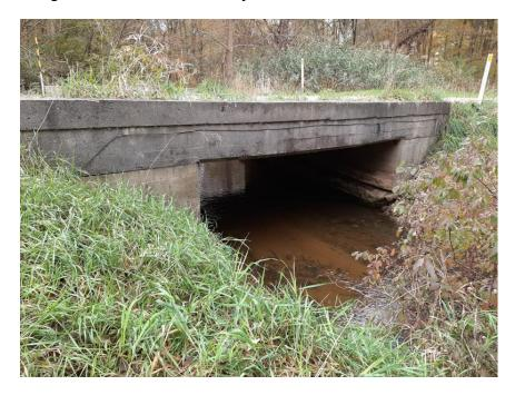
From the 2021 Bridge Condition Index, Culvert C17 was recommended to complete patch repairs and place rip-rap in eroded areas in 1 to 5 years.
