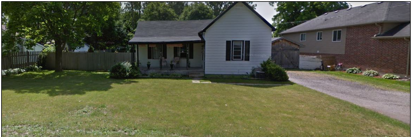
Figure 2 View of Subject Lands from Darcy Drive
